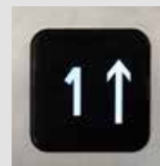
LCD DISPLAY AT LANDINGS
